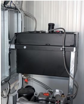
Serbatoio gasolio Fuel tank
